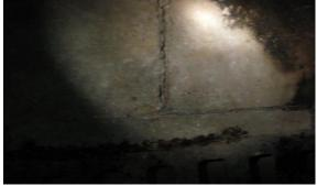
Crack in firebrick and mortar joints should be repaired.
