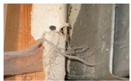
Asbestos covering noted on supply heat duct
